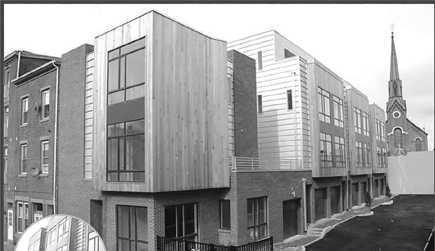
333 Green Street Townhomes located in Philadelphia, PA
