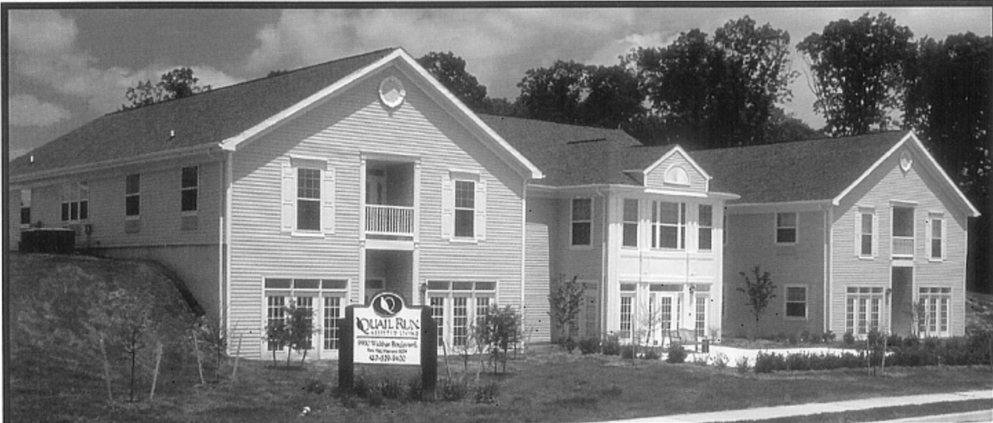
Administrative Building of the Quail Run Assisted Living Campus in Perry Hall, Maryland.
